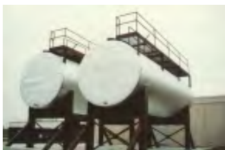
Figure 60: Horizontal tanks including concrete-lined tanks.
