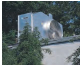
Figure 36: Fluid cooler cross flow with self-contained sump.
