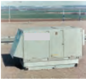
Figure 11: Small rooftop air handling unit.
